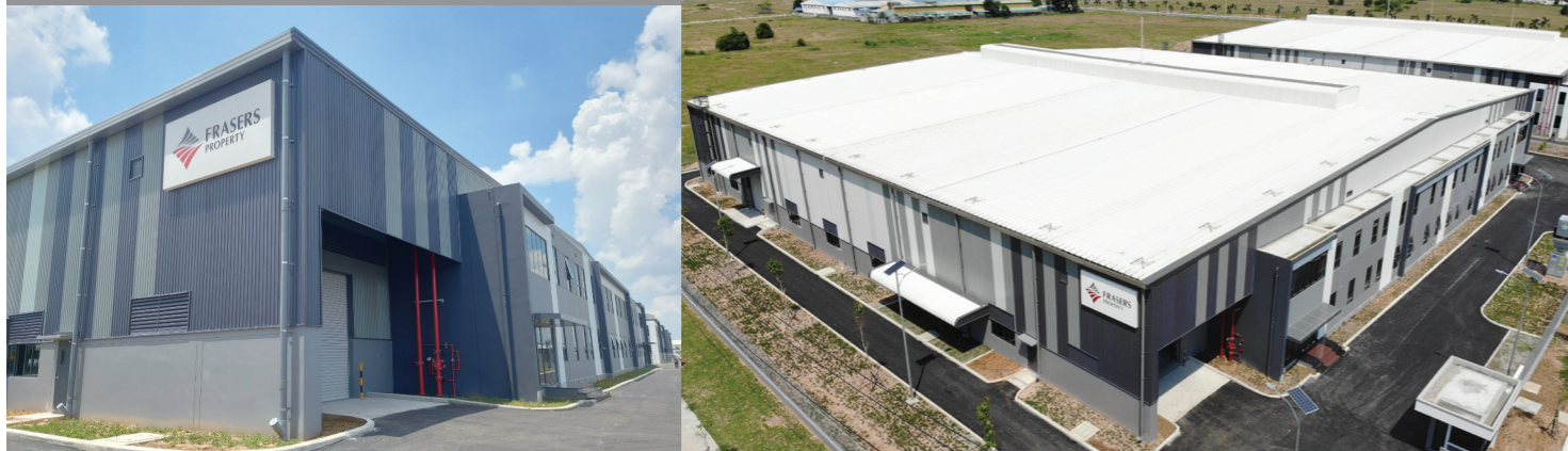
Modern factories with excellent infrastructure and amenities.
